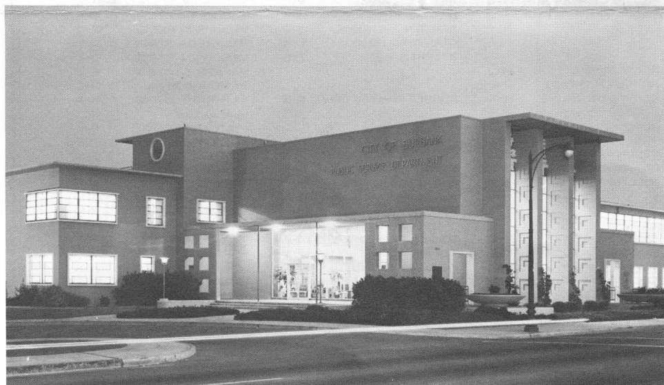
Burbank's municipally-owned utility system produces ample electric power and water for more than 34,000 homes and 400 industries.
