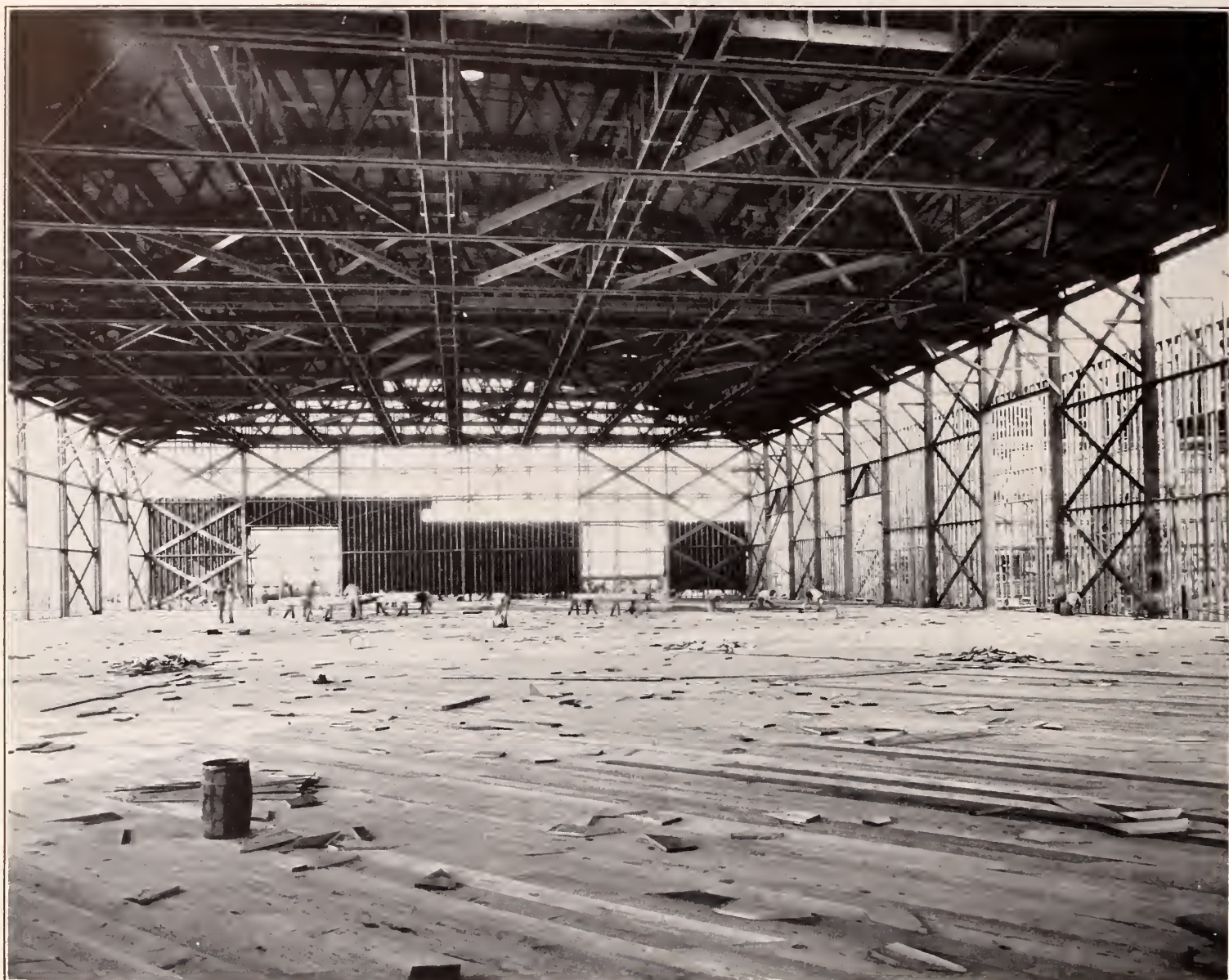
Some conception of the vast area and height of the four stages at the First National Burbank studios may be gained from this view of one of the stages under construction. The floors are so solidly built that trucks may be driven in on them with materials
