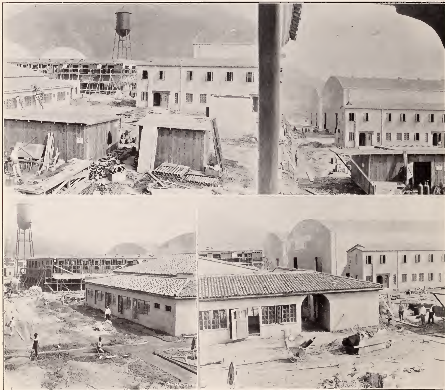
Views of the $2,000,000 First National studios at Burbank under construction, including the dressing rooms, the cutting and projection rooms, the carpenter shops and the four dark stages, which may be seen in the background of all four pictures, showing how all of the departments are grouped around the stages
