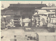
8. Giant machines like this 200-ton stretch press form bars and sheets of metal into tough airplane parts. New airplanes use strong aluminum alloys and stainless steel.
