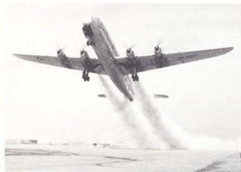
Six JATO bottles installed in Model 89's wing roots boosted mammoth plane's rate of climb.
