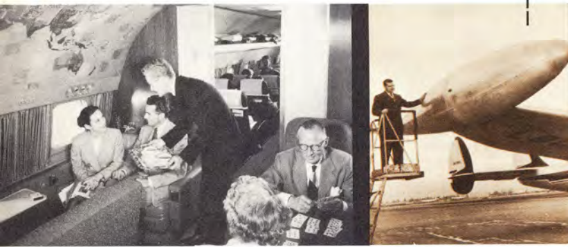
Compartments divided luxurious Model 1049C cabin at left above. At right, C. L. Johnson checked tip tank added to ocean-hopping 1049G to give longer range.
